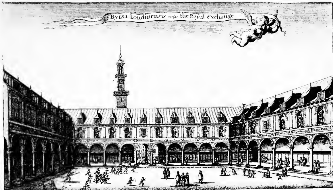
THE ROYAL EXCHANGE. INTERIOR, FACING SOUTH. 28.
